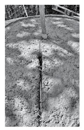
FIGURE 21.3. First thermocouple in place in subfloor; it will be cemented into a hole drilled in a hearth brick.
