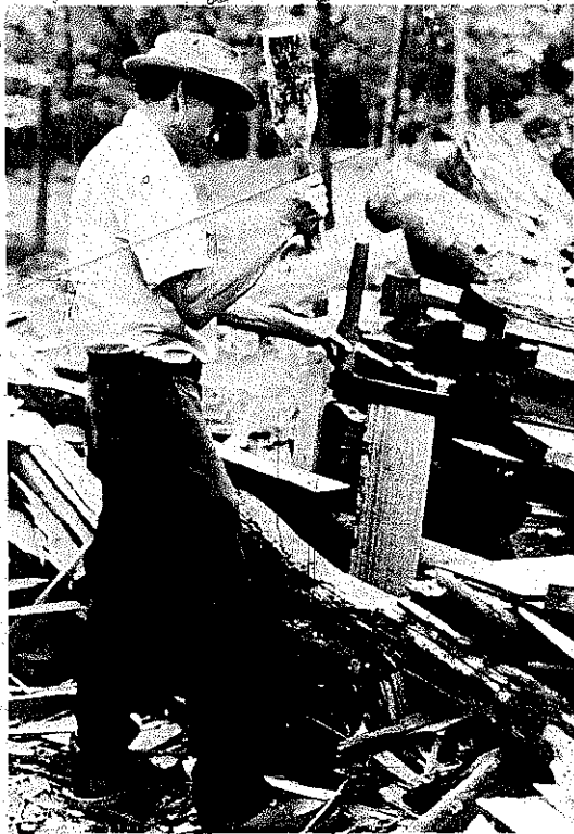
PLATES 111-113 Harley Rogers, demonstrating how to split, or rive, shingles—splitting the “bolt” which will then be split into shingles.
