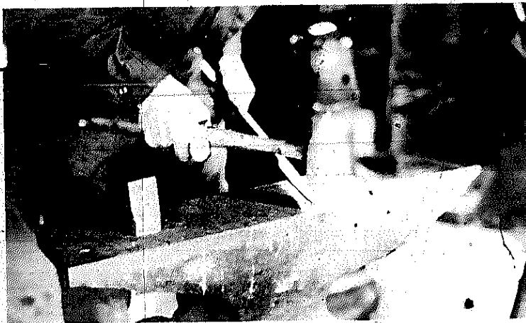
PLATE 63 Finish drawing out the point by hand.
