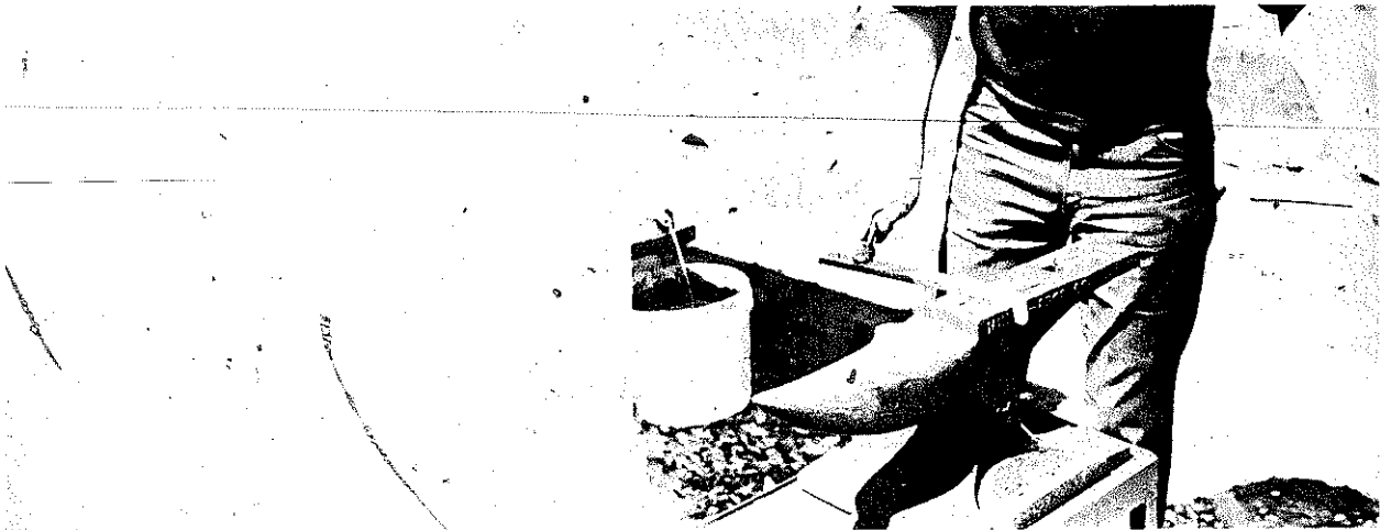
PLATES 126-127 Forming the heel caulk.
