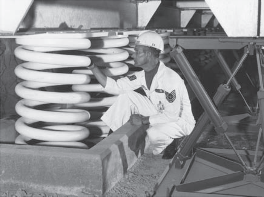
A technician checks one of NORAD's nuclear blast-resistant shock absorbers, about 1960
