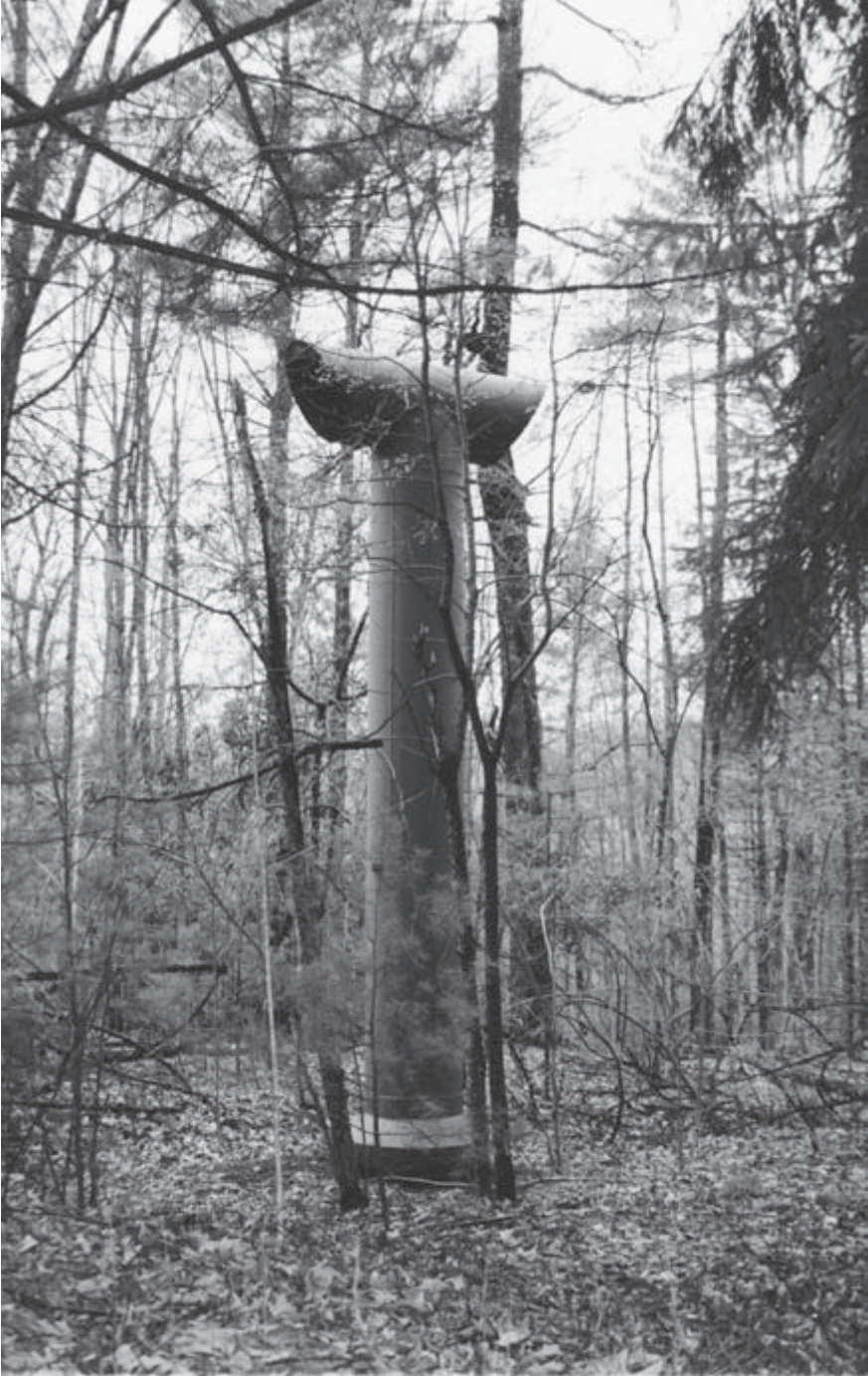
Air intake valve, Congressional Relocation Facility at the Greebriar Hotel, West Virginia
