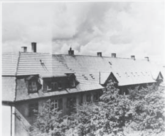
Photo 9 - Partial burn-out of row house construction. Note separating unparapetted fire walls.
