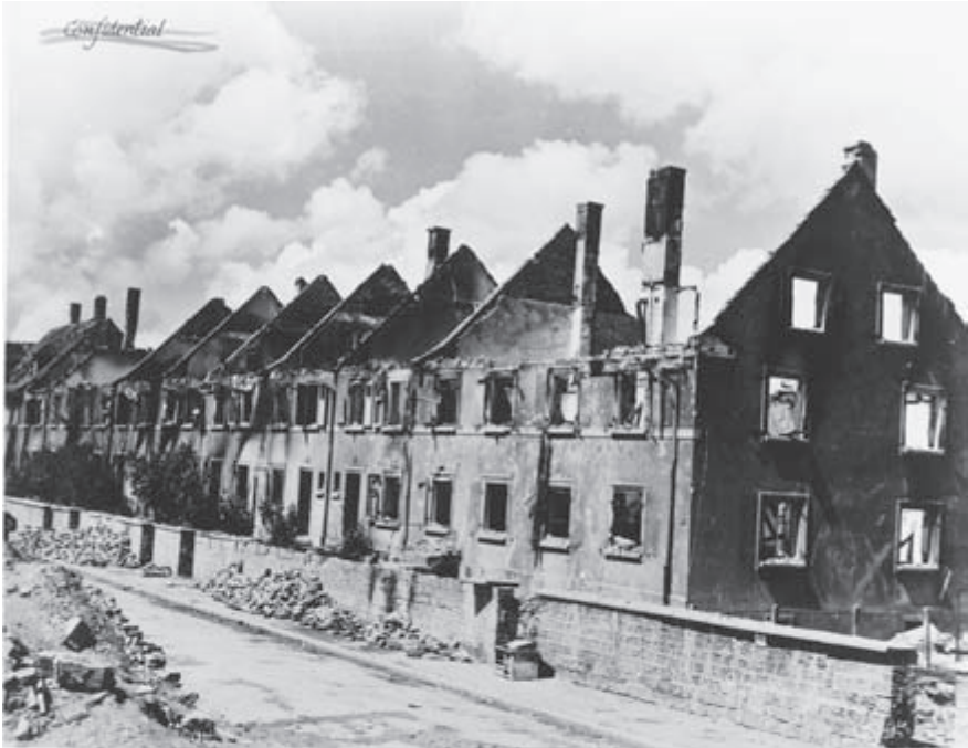
Photo 9 - Partial burn-out of row house construction. Note separating unparapetted fire walls.
