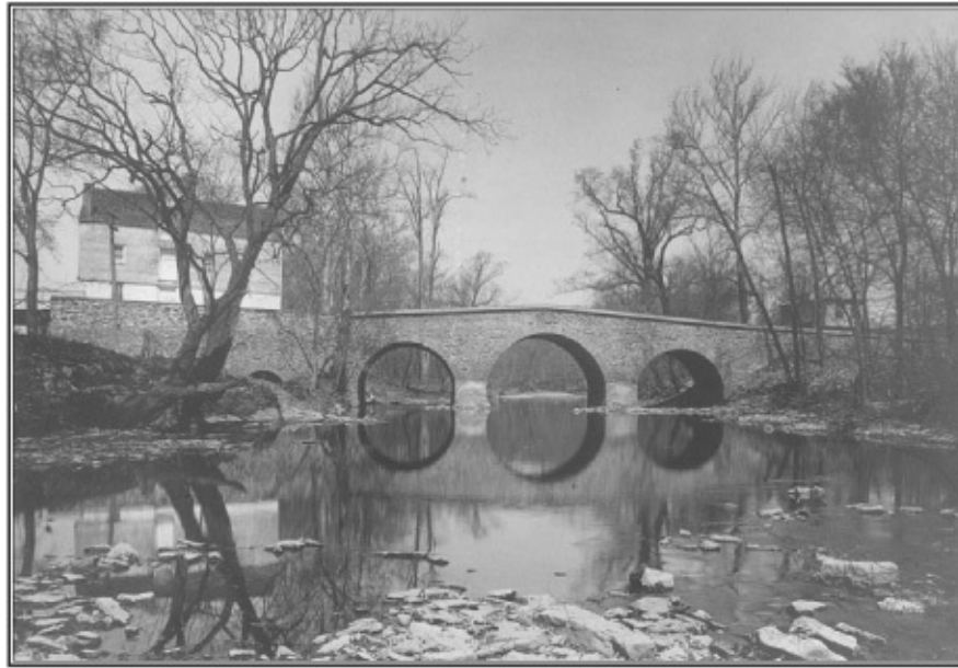
The Old Bridge over Stony Brook on the Quaker Road, a nineteenth-century photograph. This structure still stands today. Historical Society of Princeton.
