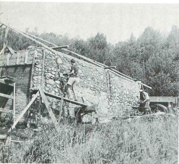
We were always building. Above, I am joined by our neighbor, Jack Lightfoot, pointing the stonework on the wall of the garage. At right is the hand-turned cement mixer, and below is the view towards Pinnacle Mountain from the sand-pit site of the stone cottage we built together in 1938.
