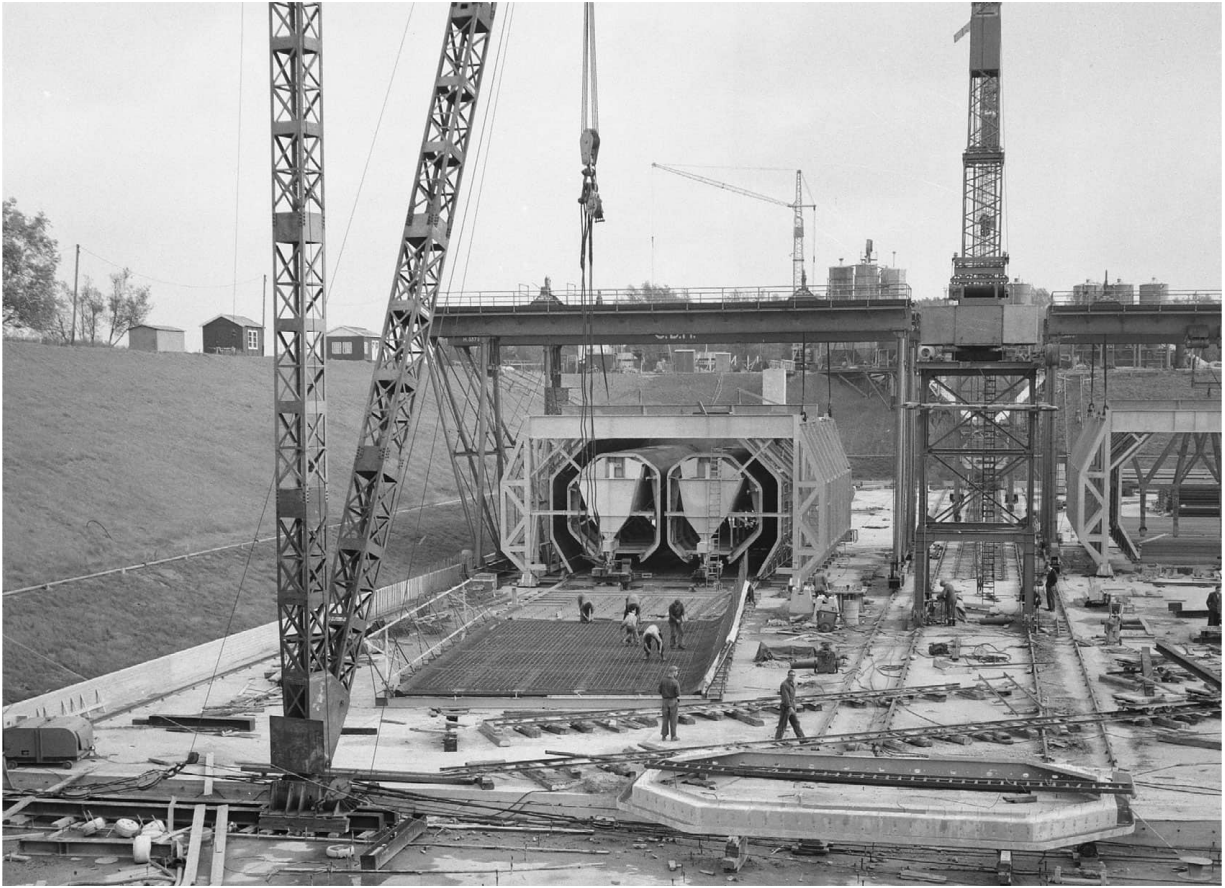
Building the first Metro line in the Netherlands took over seven years – and when it opened in 1968 it was then one of the world's shortest lines. As with anything below the water table in this country, construction was extremely expensive and time consuming. This 1961 photograph shows construction of the tunnelled sections on dry land.
