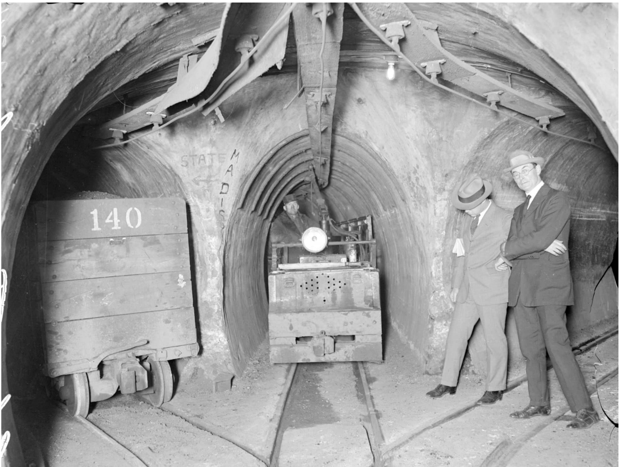
Running beneath the city's grid of perpendicular streets, the Chicago Tunnel Company's multiple freight lines had many junctions like this, photographed in 1924.
