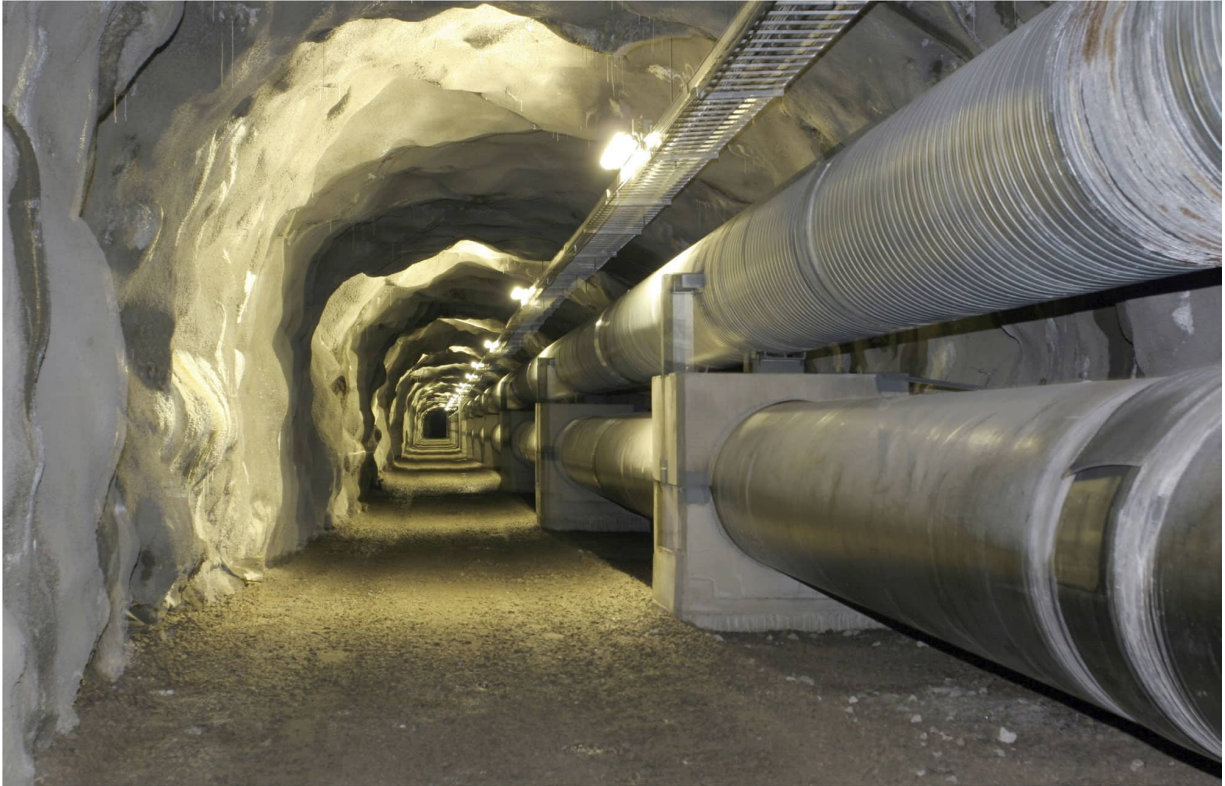
This tunnel was constructed as part of Helsinki Energy's switch to bio fuel processing. It is 30–60m (98–197ft) deep and runs for 12km (7.5 miles).
