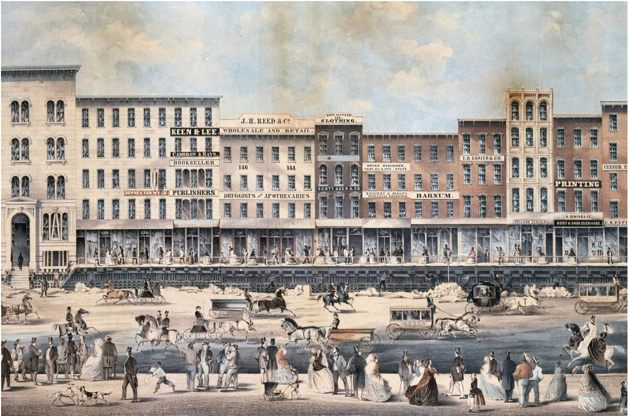
1857 illustration of the Raising of Lake Street on hundreds of jackscrews. An entire city block of 98m (320ft) was elevated in one go.
