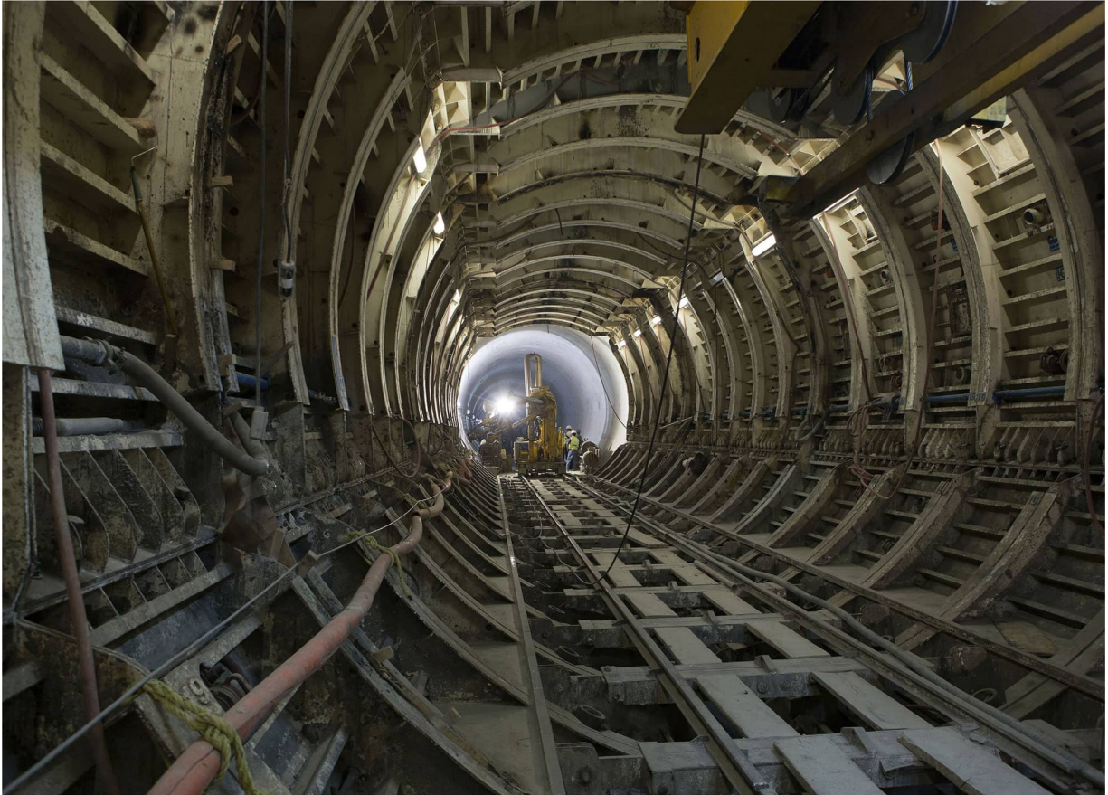
At 8.7m (28.5ft) in diameter, the controversial Tunel Emisor Oriente (or Eastern Discharge Tunnel) runs up to 200m (656ft) beneath Mexico City and took four years to build.
