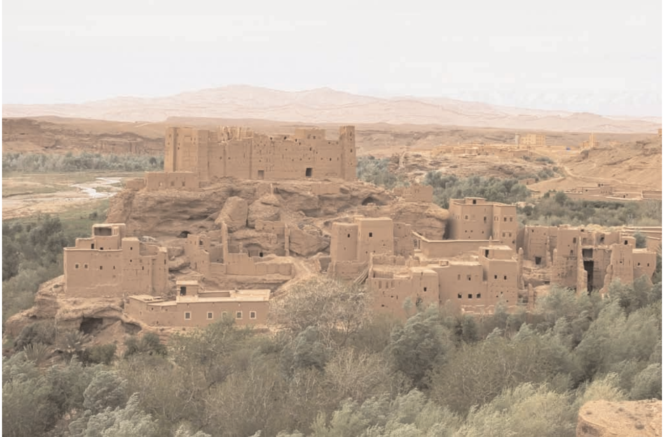
The homes in this Berber village in Morocco are made of mud and straw, a combination that, when it hardens, becomes a sturdy building material. In the hot desert climate of the region, the mud homes stay relatively cool. (Tariq Dajani/The Image Bank/Getty Images)
