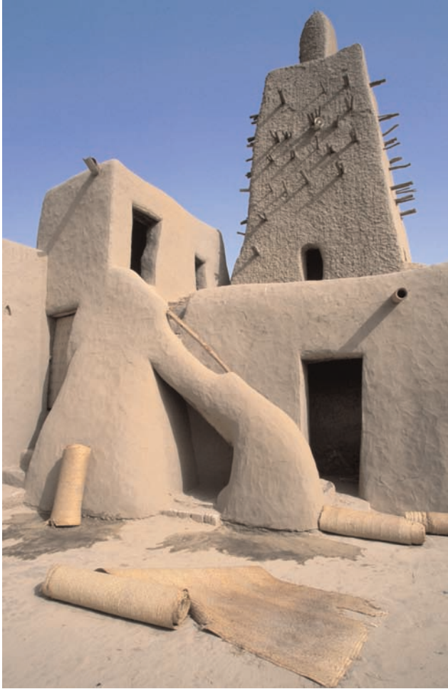
This close-up of the Djingareyber Mosque in Timbuktu highlights the texture of the mud walls. The wooden projections on the tower function as handholds for those who must reapply the mud after each rainy season. (Ariadne Van Zandbergen/Lonely Planet Images/Getty Images)
