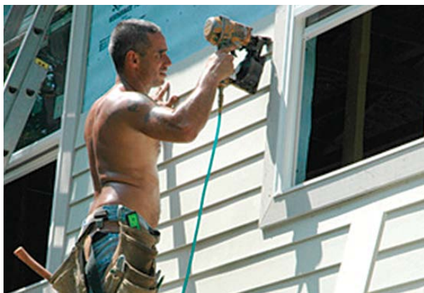
September 1, 2006. After all the trim was set in place, it took two days to wrap the building in HardiePlank siding with a 5-in. reveal.
