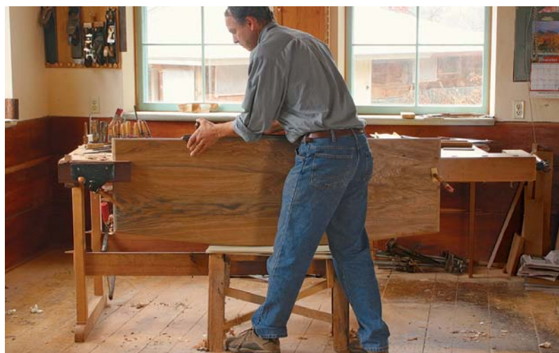
Steady a wide panel. A sawhorse provides support underneath, with the opposite end clamped to the bench apron.
