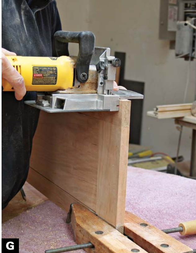
CLAMPS HOLD THE CABINET SIDES on edge, making it easier to cut the biscuit slots. Offset the biscuit location so that the front and back are inset \frac{1}{8} in. from the sides.
