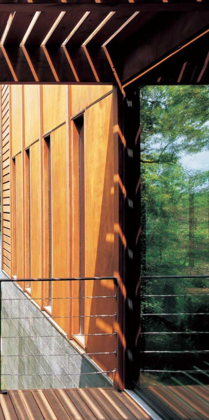
△ This modular porch looks as if it could slide in and out of the cottage like a drawer. The exterior board-and-batten siding and the open slats direct cooling breezes into the living room.
