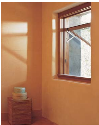
△ The interior cottage walls are clear-finished birch plywood that shimmers in the light. Operable wood casement windows are set deeply into the straw-bale walls for maximum light and minimum glare and heat gain.
