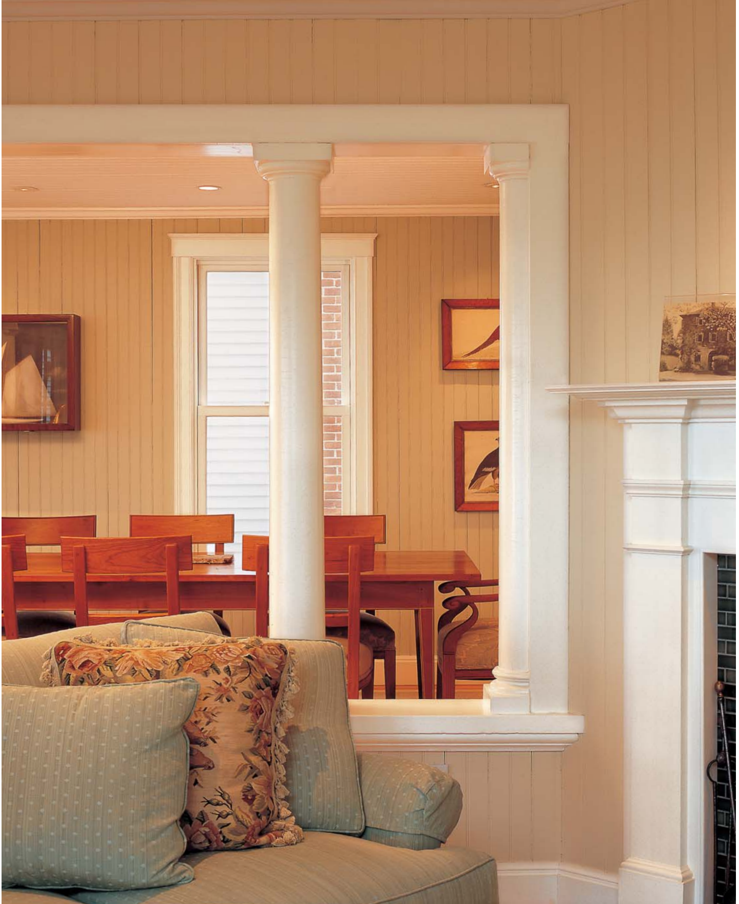
△ Colonial Revival columns and a transfer beam replace the support originally provided by a bearing wall that was removed to open up the dining room. Simple wood picture frames match the color and tone of the dining set.
