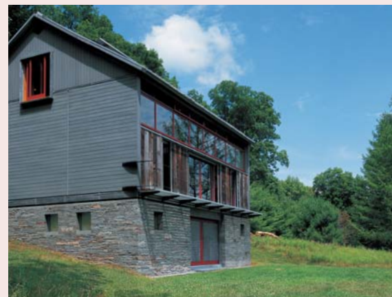
△ Bank barns, typical of the Pennsylvania barn building tradition, often have stone bases to wick moisture away from the wood siding. These original “split levels” provide easy indoor-outdoor access for sites with noticeable grade change.
