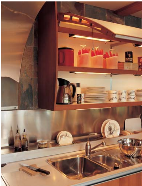
△ The graceful-looking cupboard door is constructed like a lightweight airplane wing, with fabric stretched over a light metal frame. The entire door can be removed, submerged in water and washed.
