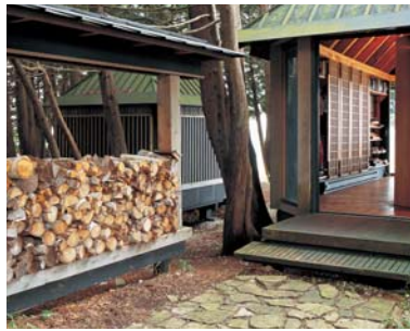
△ The building materials of this Michigan cottage and small guest cottage—iron, stone, and wood—were drawn from the abundant natural resources of the area. The steeply sloped roofs easily shed the heavy winter snows.
