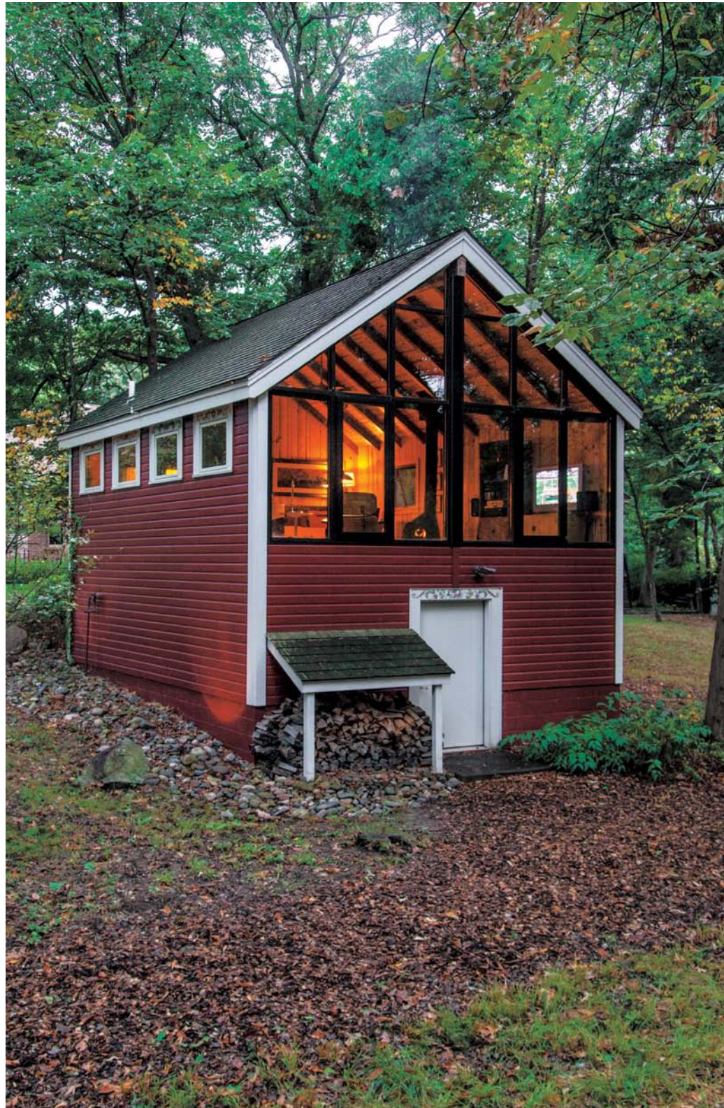
RIGHT An industrial glass curtain wall has replaced the gable end of the barn.
