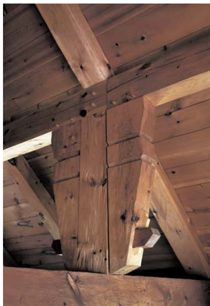
The roof load on the rafters is transferred to the purlins, which bear on the queen post, which transfers the load to the cross ties.
