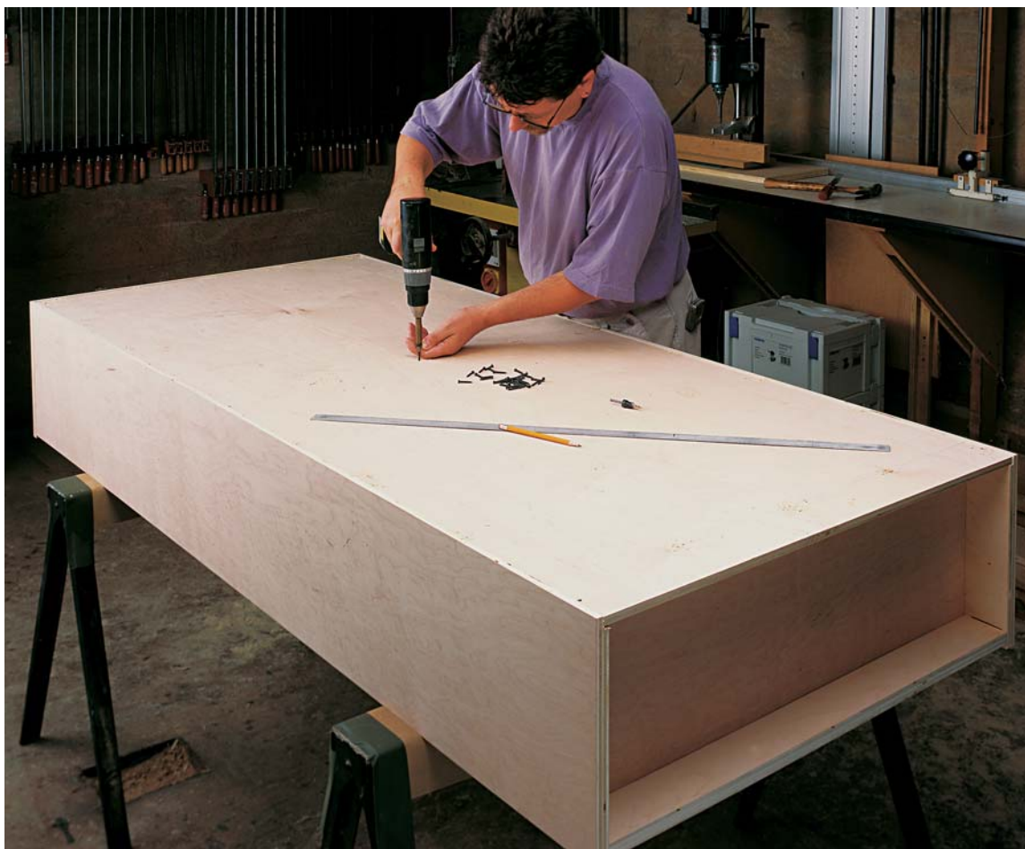
Photo I: Screw on the back with trim-head screws. These have very small heads that make them ideal for attaching the back along the thin rabbeted edge.
