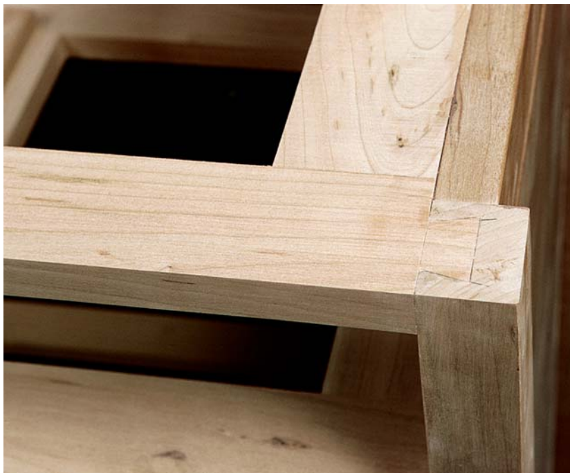
Photo M: A large dovetail cut on each end of the top drawer and back rails join them to the posts. This traditional joinery captures the rails in the posts.
