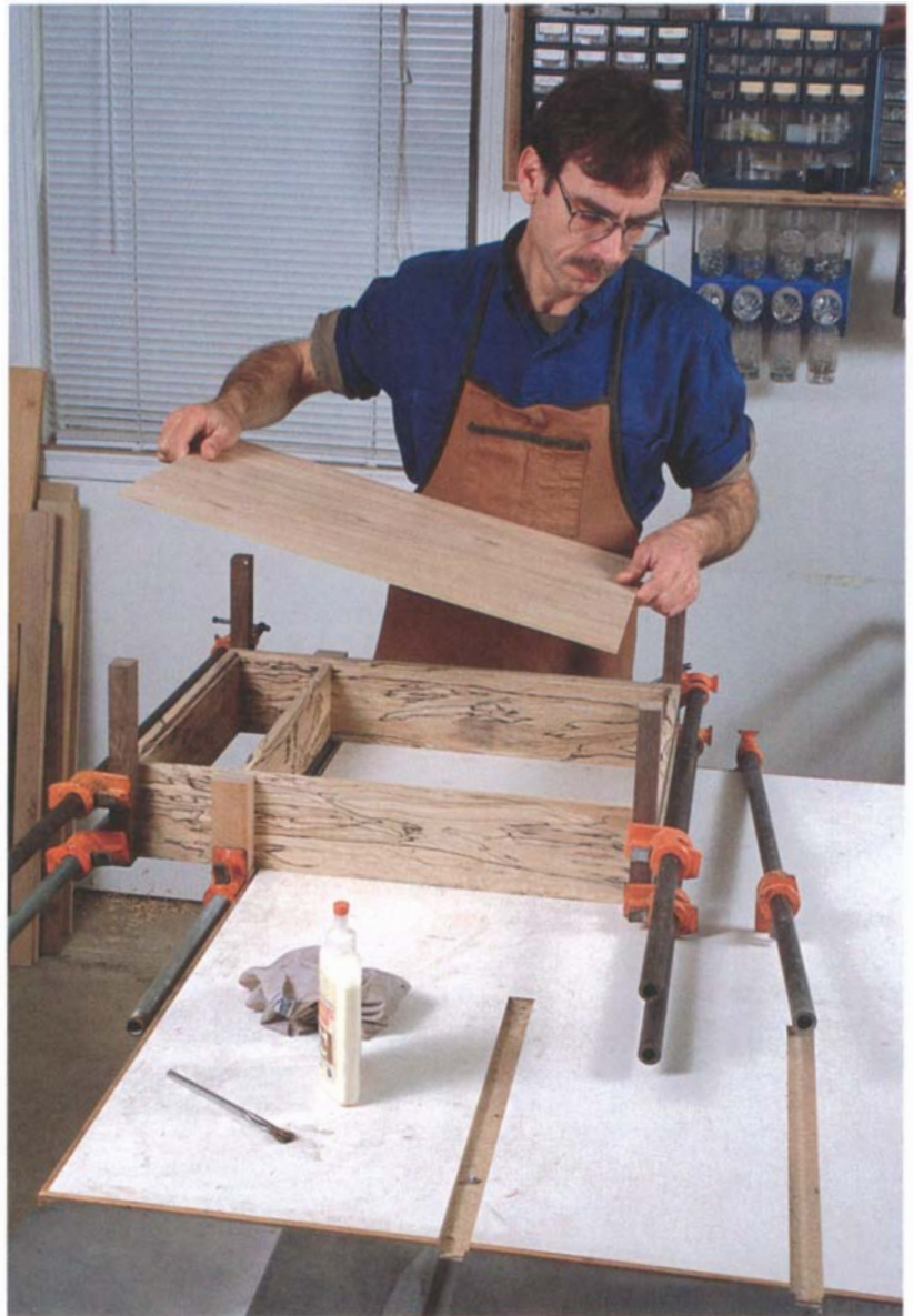
PHOTO D: Before gluing up the case, do a dry-fit to check your joints and rehearse your clamping procedures. The back, cut to fit tightly in its rabbets, helps hold the case square while the glue cures.
