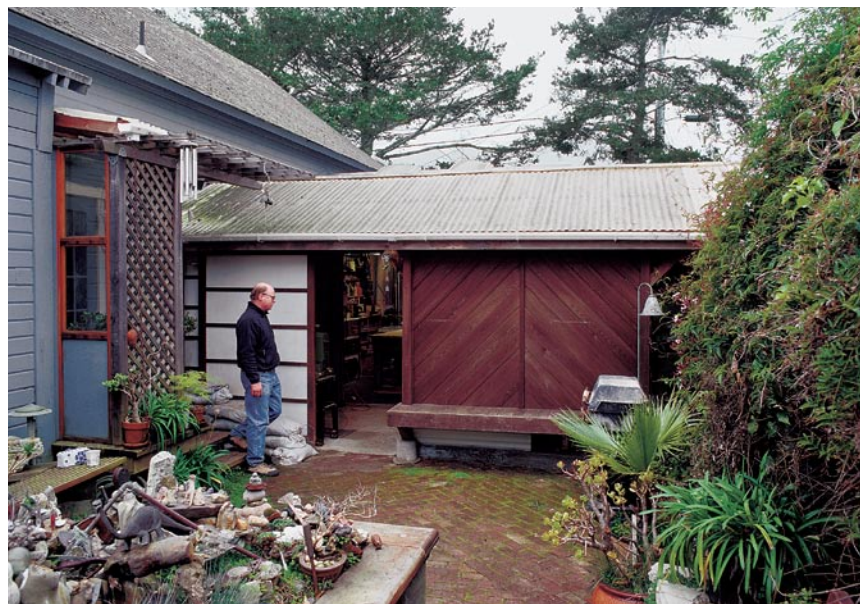
An inexpensive addition to the rear and side of Jim Casebolt's single-car garage doubled the size of his shop. By using a translucent corrugated-fiberglass roof, he gained loads of natural light as well.
