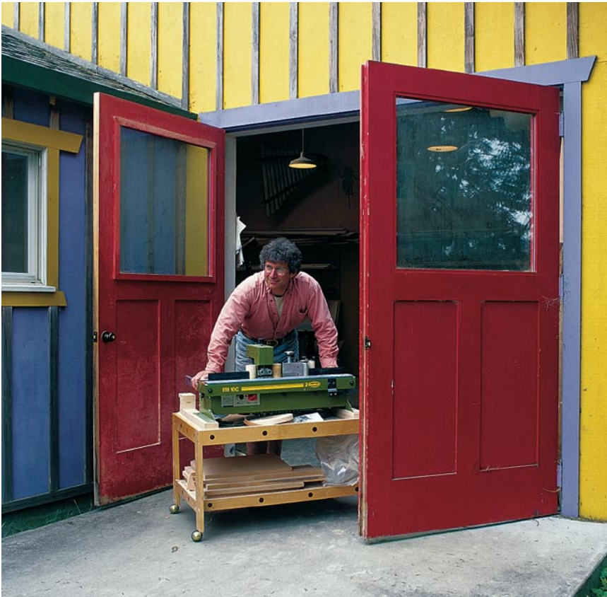
A pair of big double doors can make life in the shop a lot easier: One door provides daily access, whereas propping both doors open allows you to move large machines, materials, and projects in and out of the shop easily.
