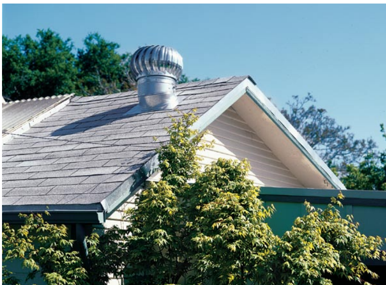
A roof-mounted turbine ventilator can use the slightest passing breeze to draw hot air from a stuffy attic or directly from your shop space.
