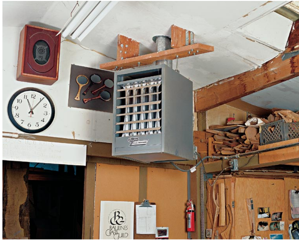
A gas-fired unit heater suspended from the ceiling can provide one of the quickest ways of heating a shop with high ceilings and a fairly large, open floor space.
