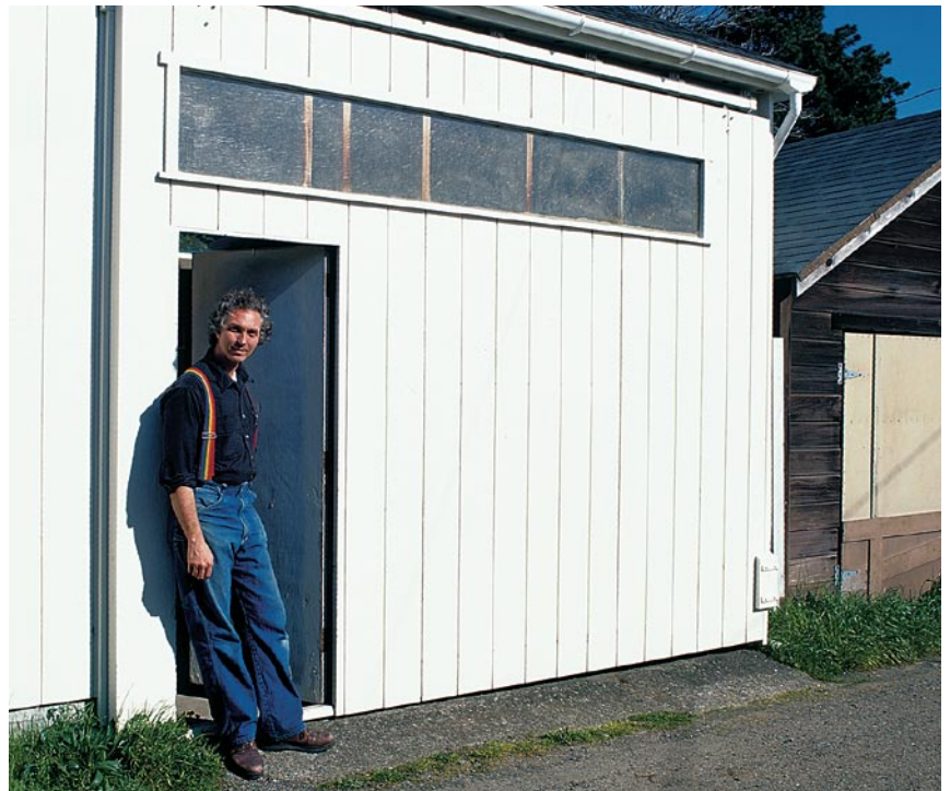
To spare the effort of moving a big sliding door every time he enters or exits, woodworker Dan Stalzer installed a standard hinged entry door directly into one end of the slider. He also added a long, translucent fiberglass-glazed window to let in natural light.
