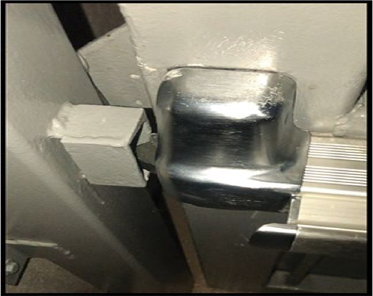
An inside view of the pedestrian gate, showing the latch and the dead latch mechanism along with the opening in the hardware allowing a hand or a tool to fit through to push the exit push bar.
