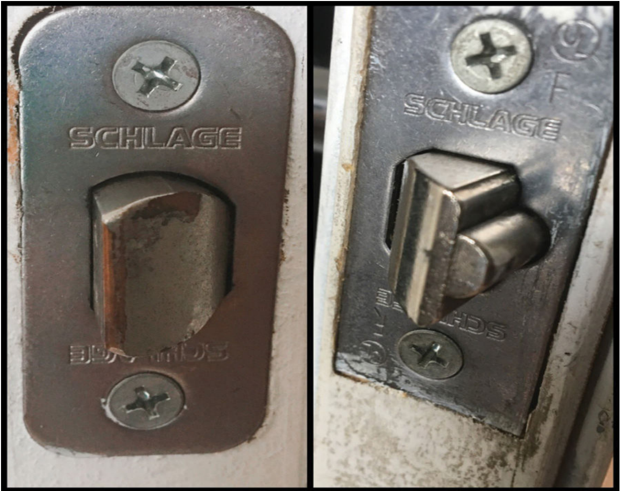
(Left) A simple latch. (Right) A latch with a deadlatch mechanism.
