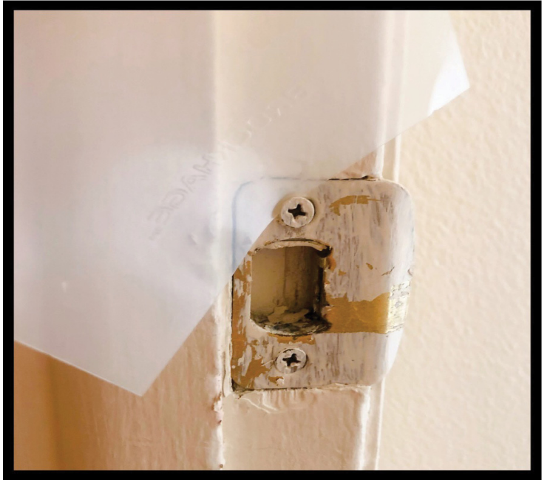
Cheap door, cheap frame, cheap latch strike plate, shitty installation. A surprisingly effective defense against shim attacks!
