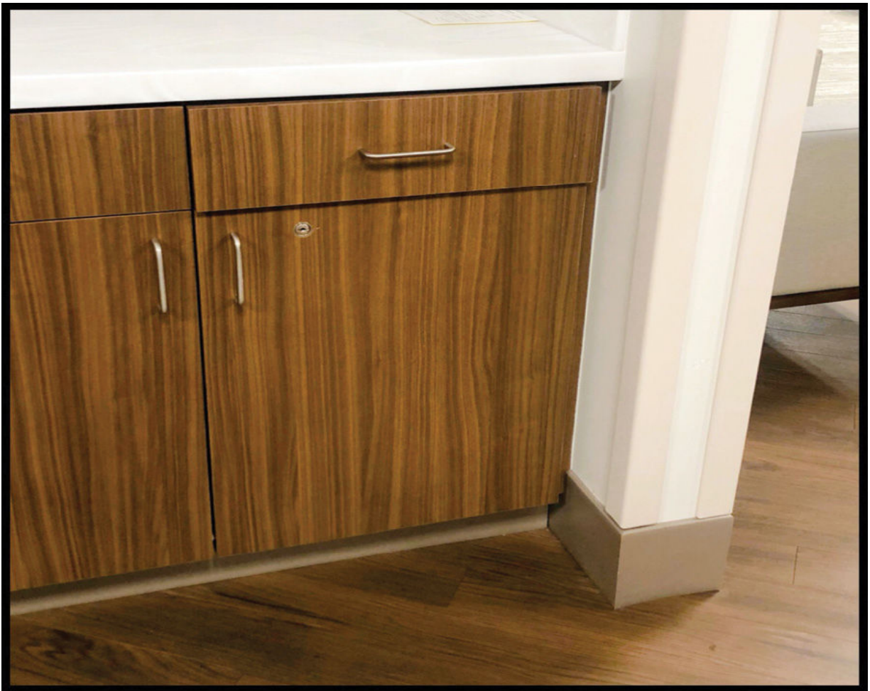
A simple locked cabinet utilizing a low-security wafer lock.
