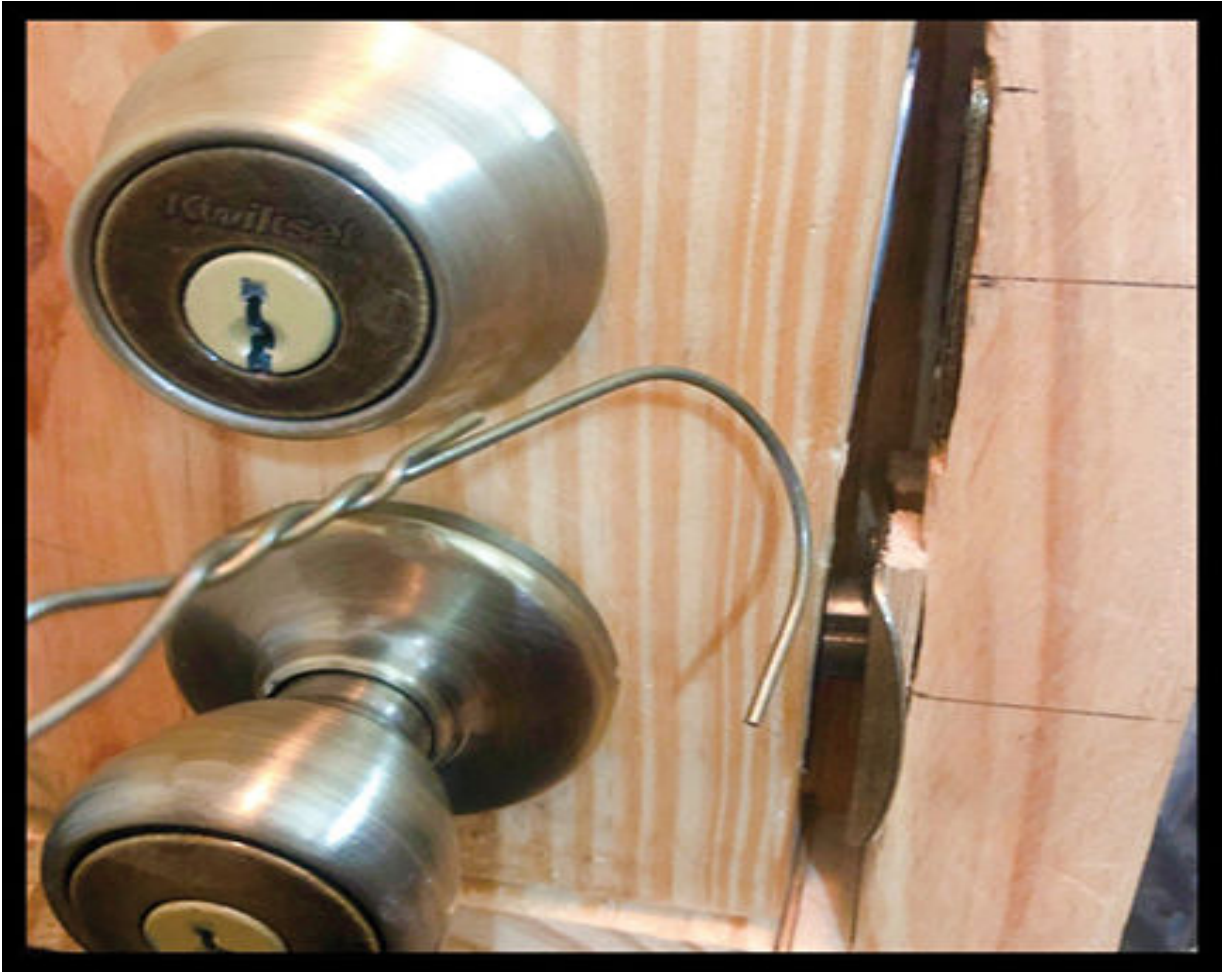
A training door with a wide gap in the door jamb. The gap makes it easy to fit tools between the door and the doorframe, which in turn makes it easy to manipulate the door latch.
