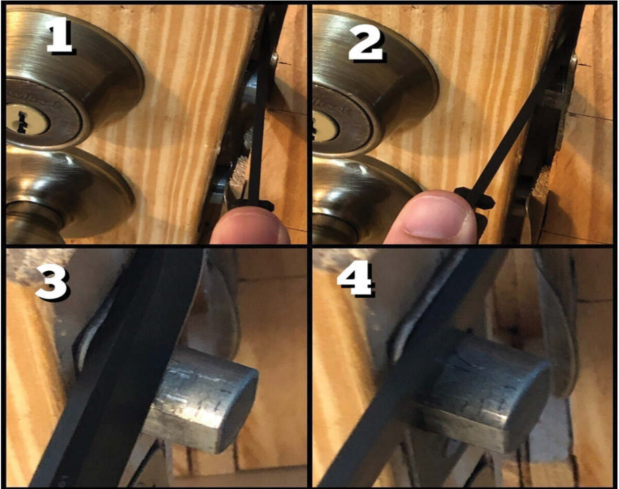
(1) A pocketknife digs into a deadbolt, close to the doorframe. (2) The knife slides toward the door, where the latch would recede to the unlocked position. (3) The knife digs into the deadbolt. (4) The knife “walks” the deadbolt in toward the door (and the unlocked position).
