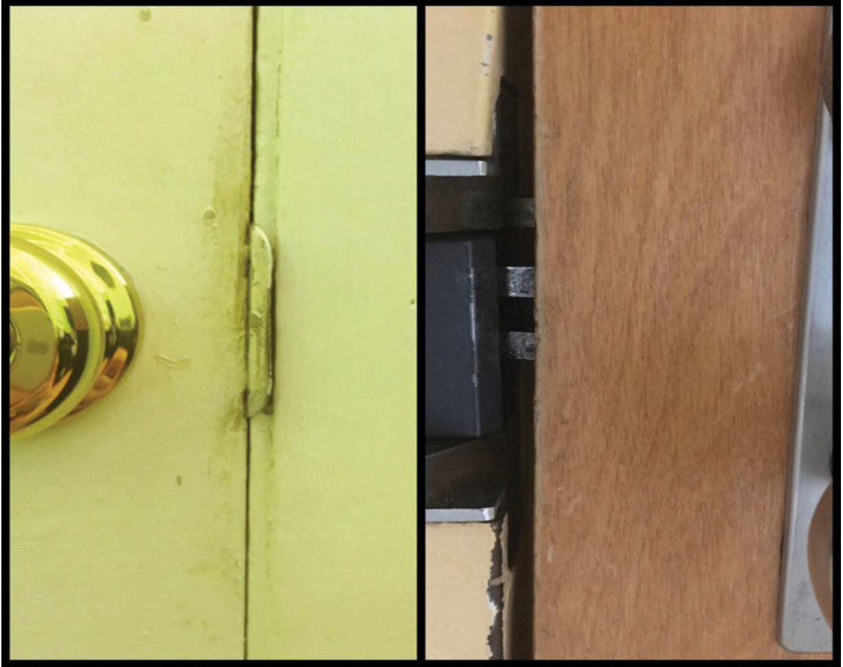
(Left) A door jamb that is very tight, making it very difficult to insert entry tools. (Right) A high-security commercial door latch with an oversized latch strike plate (improper fit) and a very wide gap in the door jamb (improper fit), allowing a successful attack with a coat hanger.
