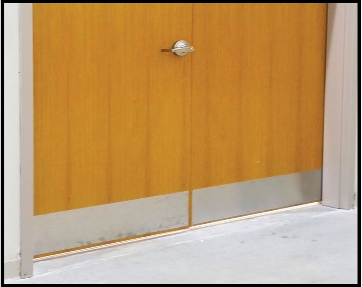
A commercial double door with a huge gap underneath, visible from far away.
