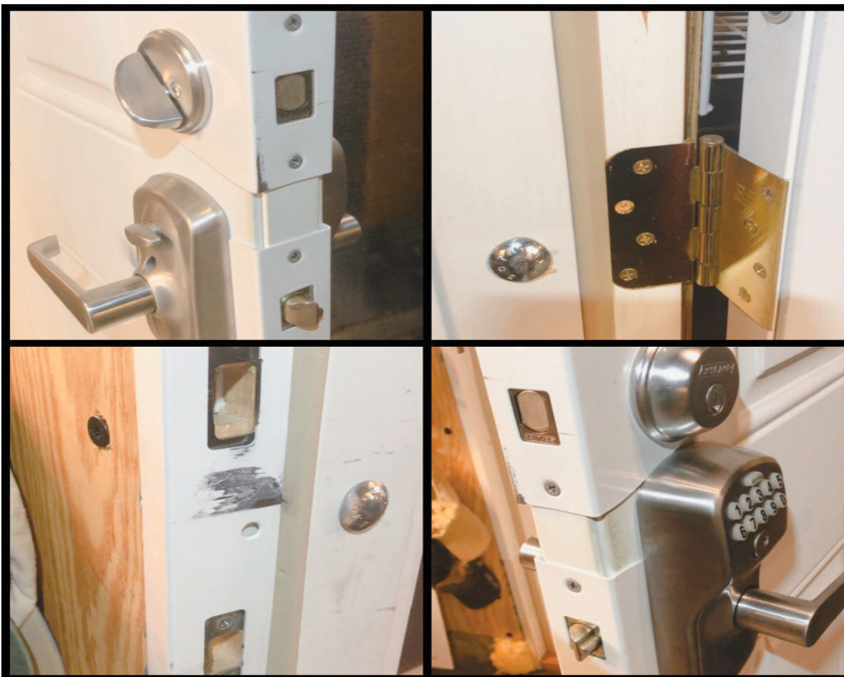
Reinforcing hardware on an interior residential basement door to prevent forced entry. Slightly costly but once installed it doesn't change the way you live your life. This is exactly the type of security upgrade I promote.
