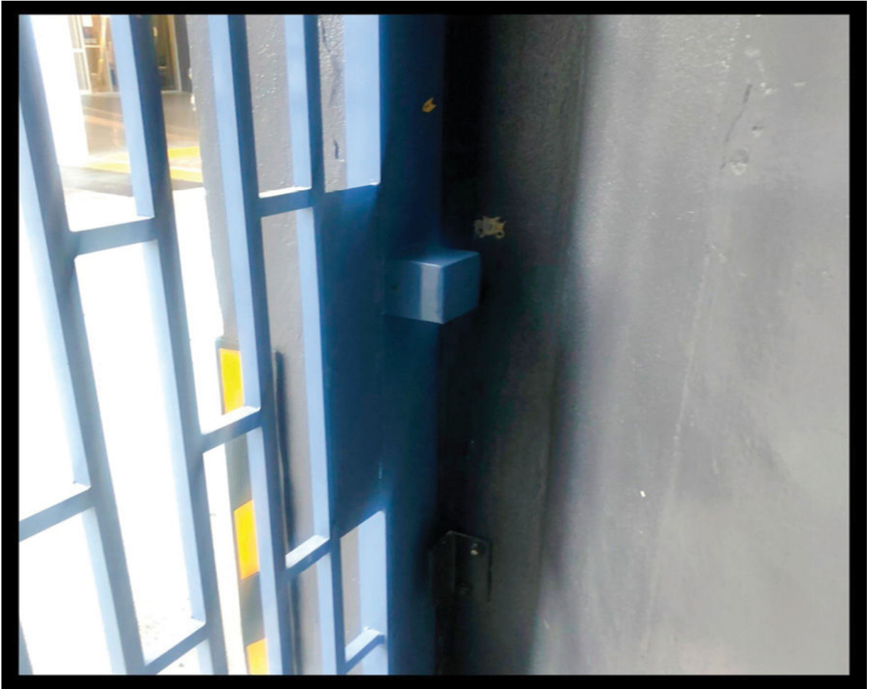
View of the inside of a gate with a low-security padlock shielded by an exterior box.
