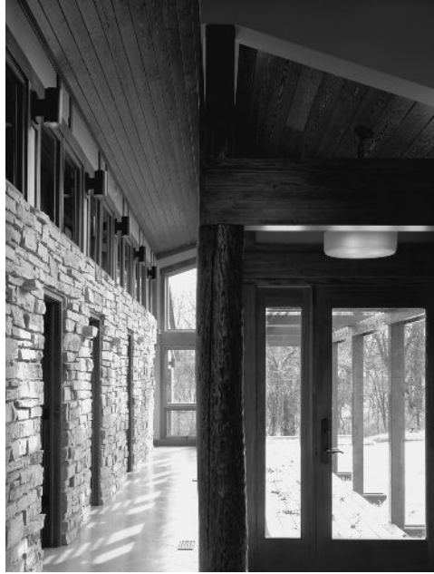
The heat-retaining interior “trombe” wall of the Lawrence home
