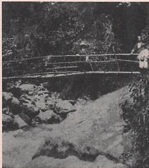
CANE BRIDGE IN THE HIMALAYA RANGE
