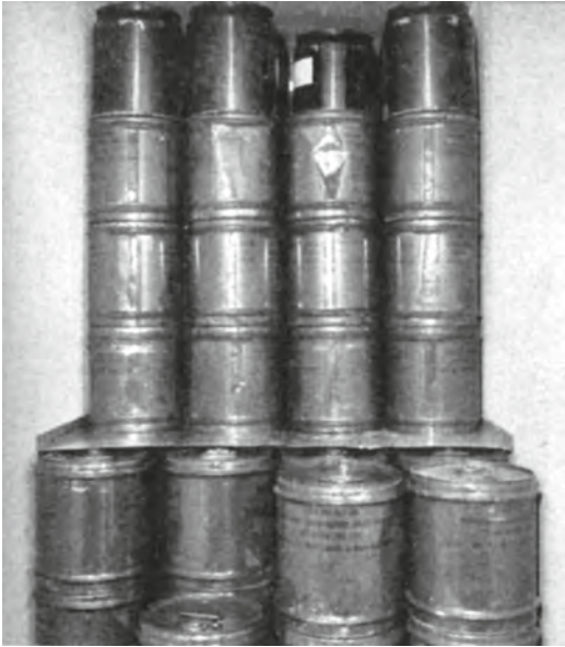
Phase Change Storage Heat Bins, design by Eleanor Raymond and Mária Telkes, at Dover Sun House, near Boston, Massachusetts, USA, 1947–52.
